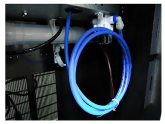
CAUTION: All connections must have the supplied locking clips installed
